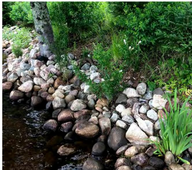
FIGURE 11: ROCK RIPRAP TOE WITH UPLAND GEOTEXTILE BAGS
